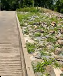
Looking up boat ramp.
