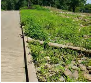
Looking up boat ramp
