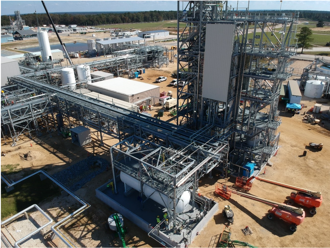
Figure 2: October 2019 Image of Thermal Oxidizer Structure During Construction.
