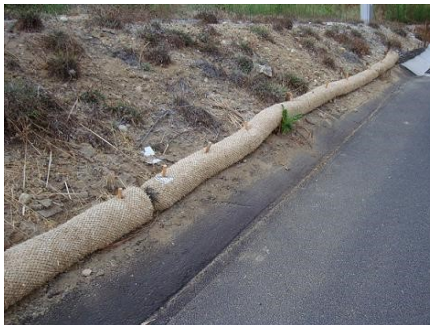
Figure 12. Example Erosion Control Measure (fiber rolls)
