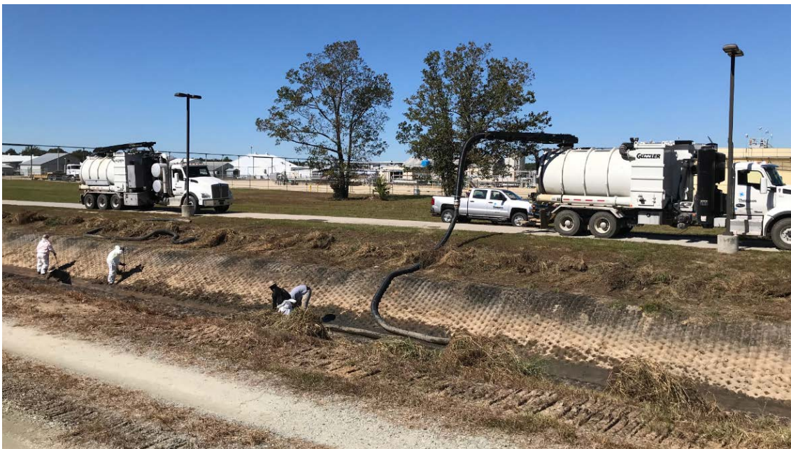
Figure 11: Sediment removal from Open Channel on October 15, 2019
